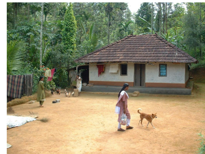
2.2. Adivasi house made of bamboo, loam and tiles
